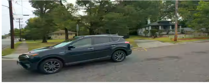
(a) Transitions from a one-way road potentially encroaching on oncoming vehicles
